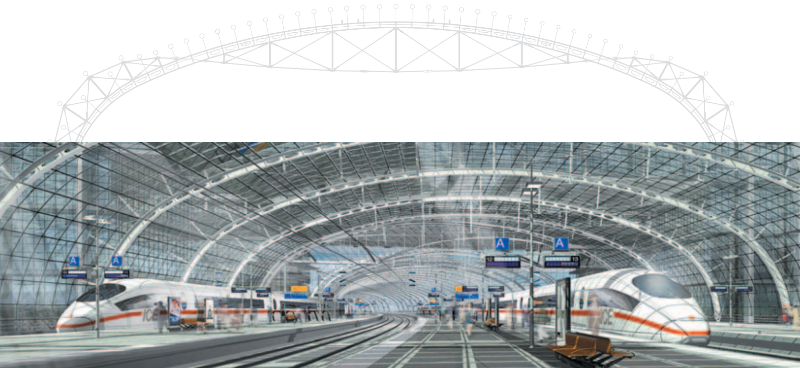
Lehrter train station in Berlin: The roof structure of Europe's largest train station spans 300 m of platforms and contains numerous ELGES spherical plain bearings and bolt systems (Photograph courtesy of Computersimulation (C) Archimation, Berlin)
