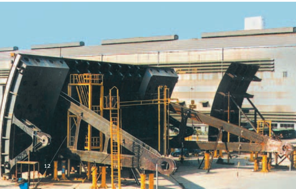
Gigantic: The flood gates in the Saemangum dam have a height of 15 meters and a width of 30 meters
