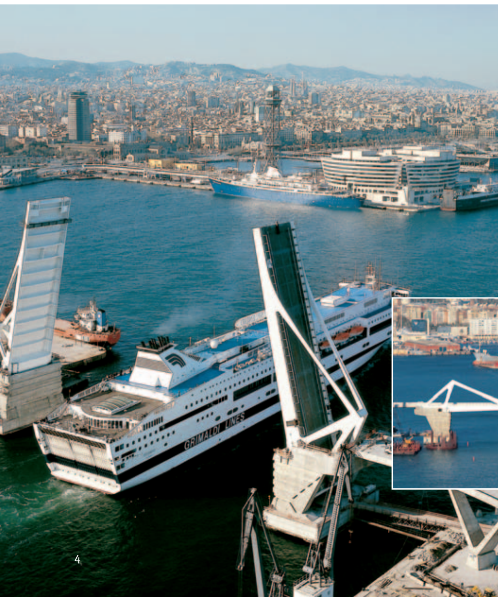
Barcelona. The world's largest double bascule bridge pivots on maintenance-free large spherical plain bearings with bore diameters of 670 mm.
