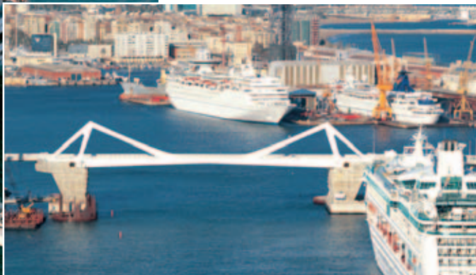
Barcelona. The world's largest double bascule bridge pivots on maintenance-free large spherical plain bearings with bore diameters of 670 mm.
