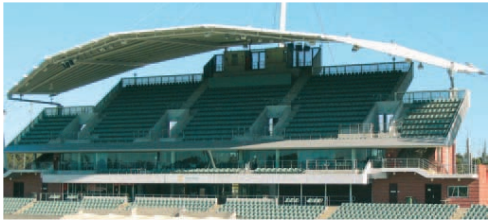
The State Hockey Centre in Sydney – all of the rope coupling points at the edge of the roof and on the masts have supports incorporating ELGOGLIDE® spherical plain bearings
