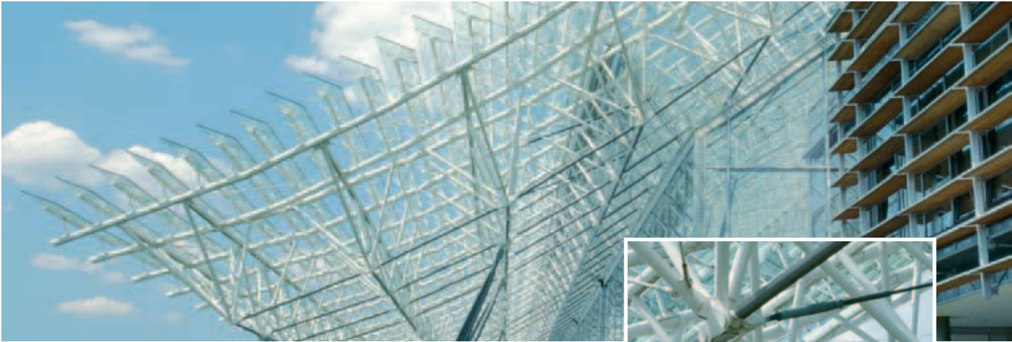
dvg building, Hanover: The roof hovers above visitors like a huge cobweb
