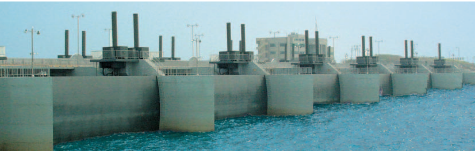
Land reclamation project in Korea – Saemangum: This dam, completed in 2001, is one of the most interesting applications for ELGES products
