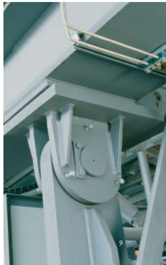
Spherical plain bearings in the supports under the platform: When raised, they allow the playing field to be moved in and out
