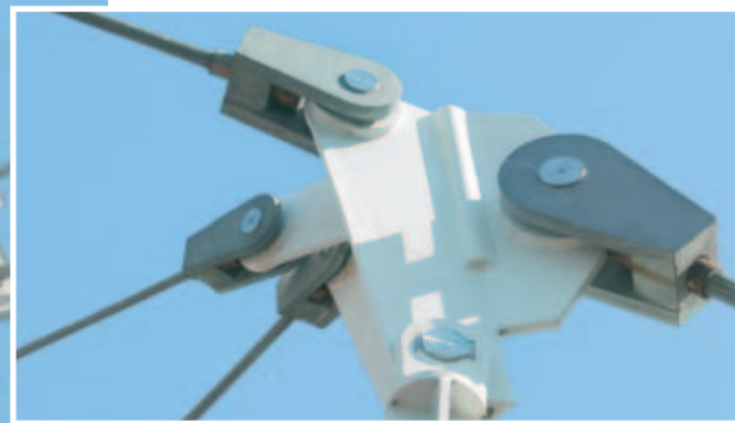
Sophisticated solutions that support extremely high loads: Rope coupling points in the roof design
